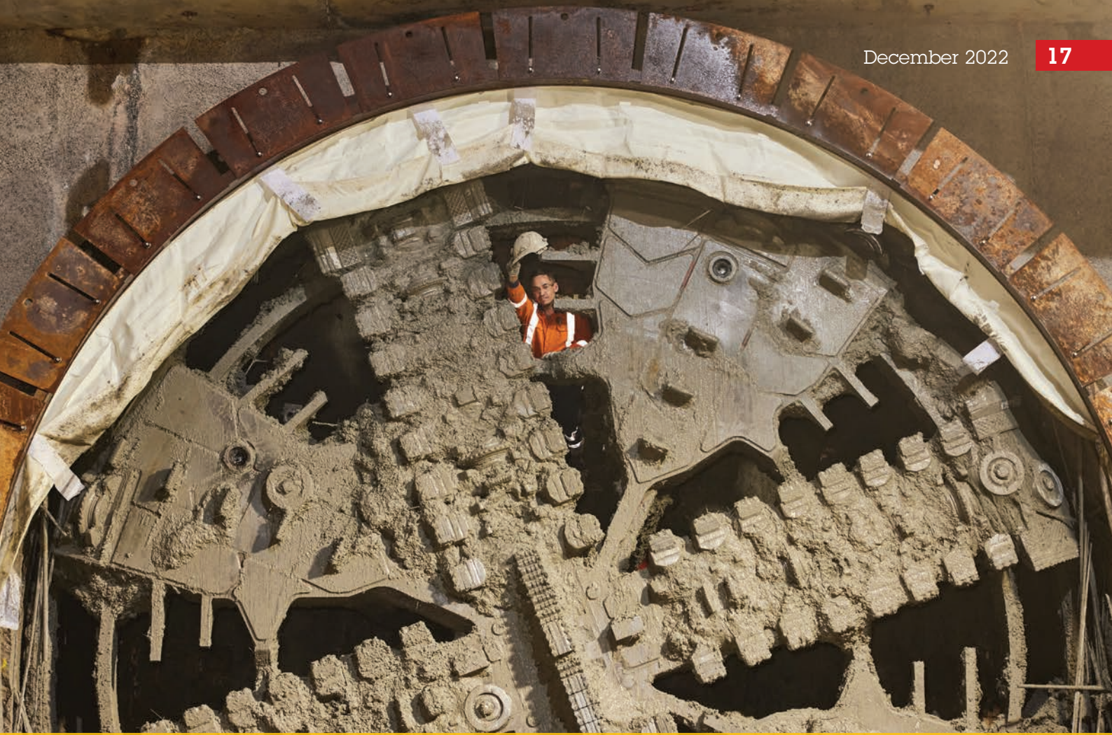
The final breakthrough and completion of tunnelling the City Rail Link.
